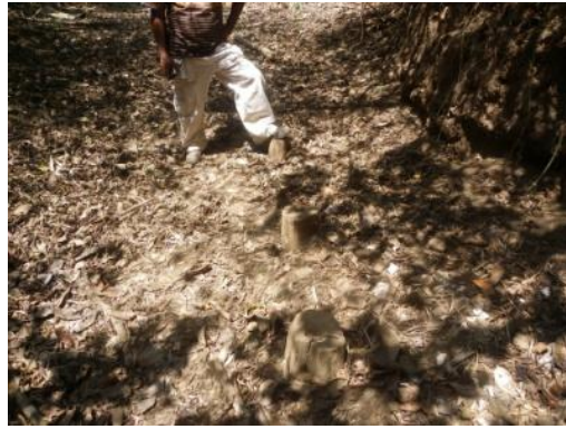
Two sets of three piles of the southern creek timber crossing
