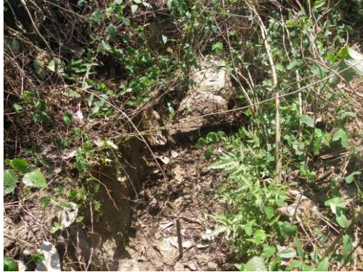
Concrete railway footing north creek crossing
