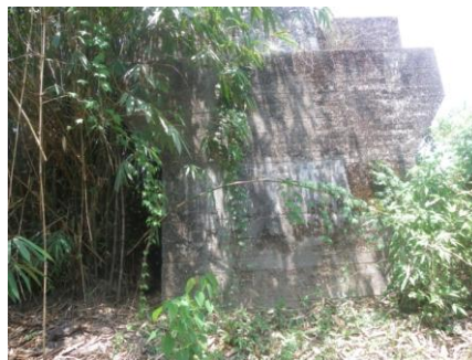
Concrete bridge pylon No. 1
