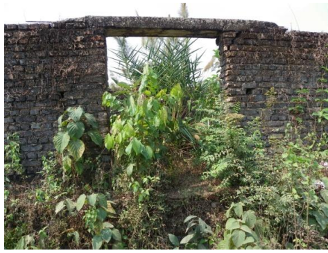
Remains of old unidentified building beside the railway
