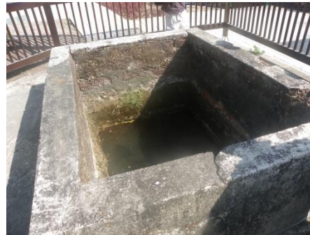
Hot springs holding tank
