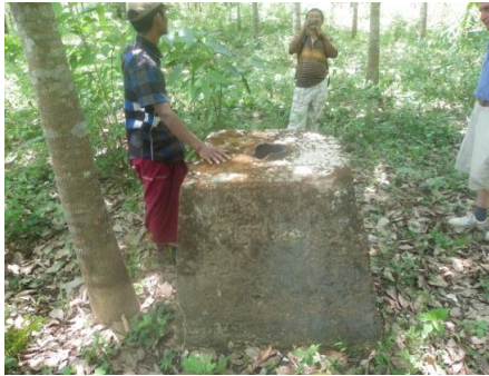
Concrete base for replenishment pipe supplying overhead locomotive water tank
