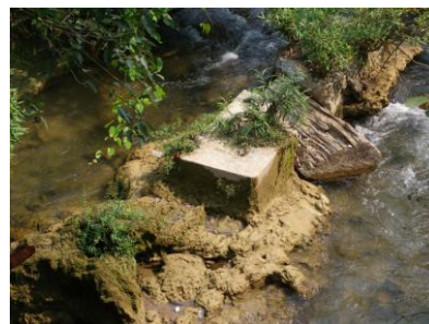
Second timber river crossing
