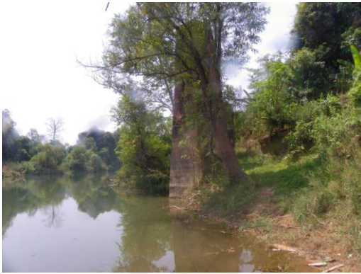
Concrete pylon north bank
