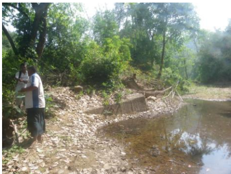
Concrete footing of timber trestle bridge crossing
