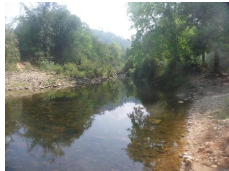
Embankment head on left hand side of river
