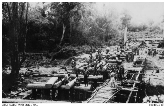
Construction of timber bridge 1943
