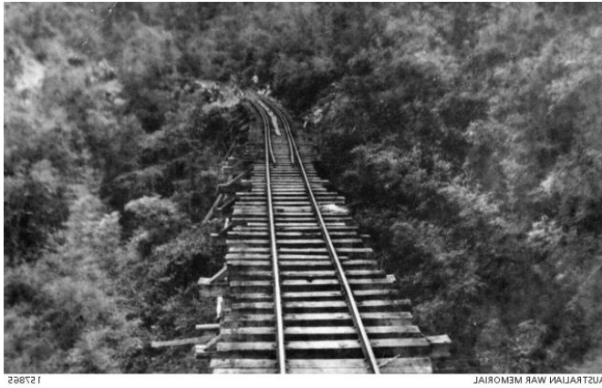
Bridge after construction
