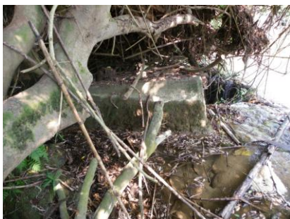
Concrete footing Zamie river crossing
