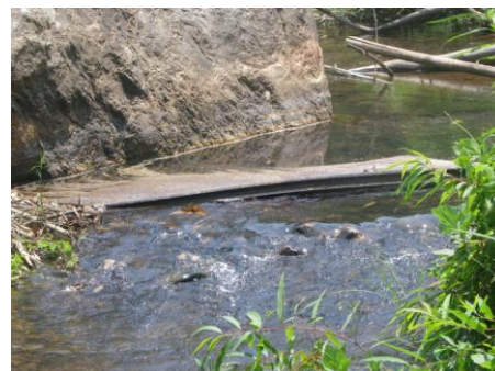
Rails at foot of concrete embankment head
