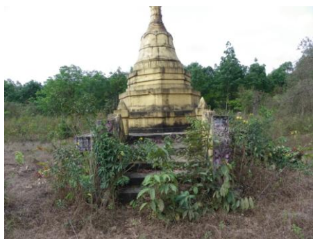
Old pagoda beside the railway embankment
