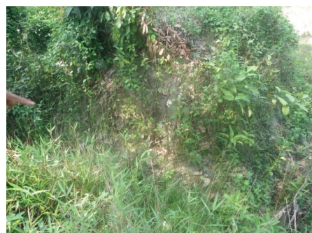
Remains of timber culvert crossing
