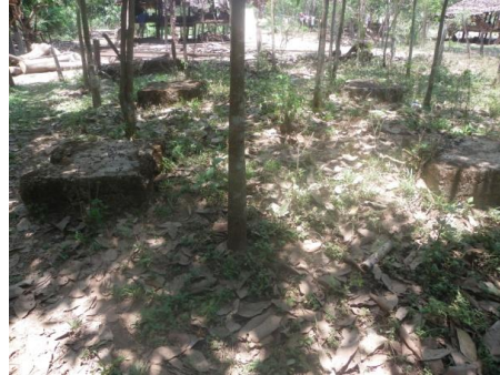
The four concrete foundations for the overhead locomotive water tank
