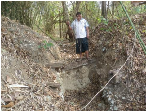
Concrete footing for timber culvert
