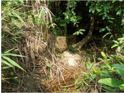
Concrete footing between Regue and Kyondaw
