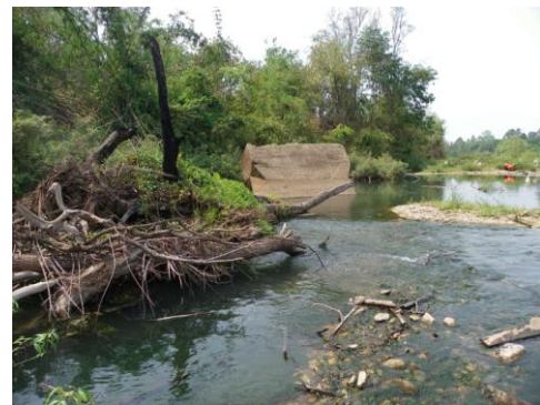
Remains of the two concrete pylons of main steel bridge as a result of allied bombing (both pylons lying on their sides)
