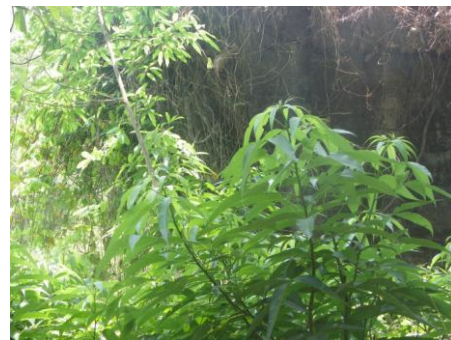
Aparaine bridge concrete pylon
