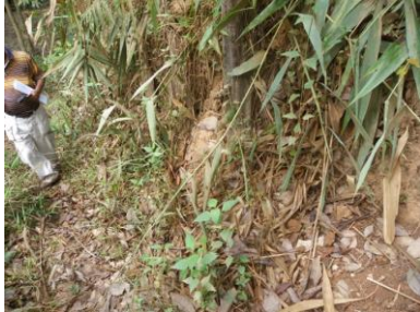
Remains of timber embankment head for timber trestle creek crossing
