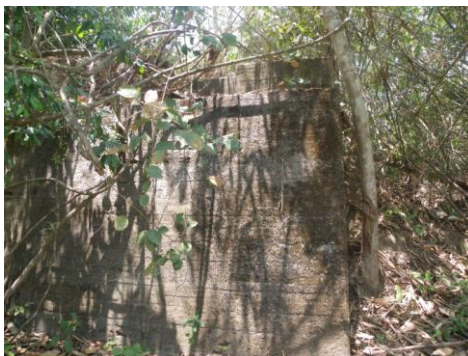
Second concrete pylon
