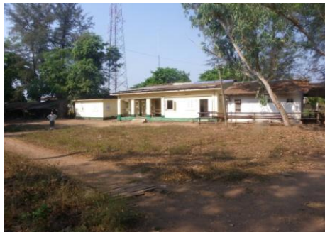
Site of train consolidation sidings (2) constructed at rear of Thanbyuzayat Station
