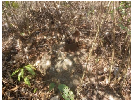
Locomotive water feeder pipe to overhead tank
